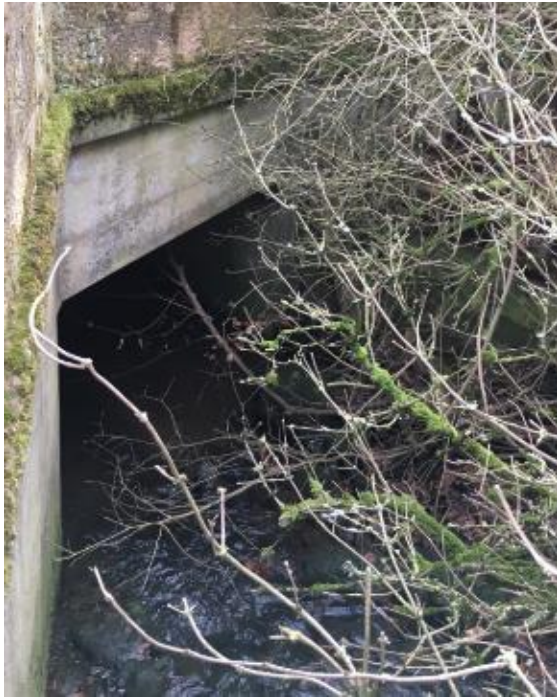
Image 10-30 – Shipperton Bridge (Inlet)
