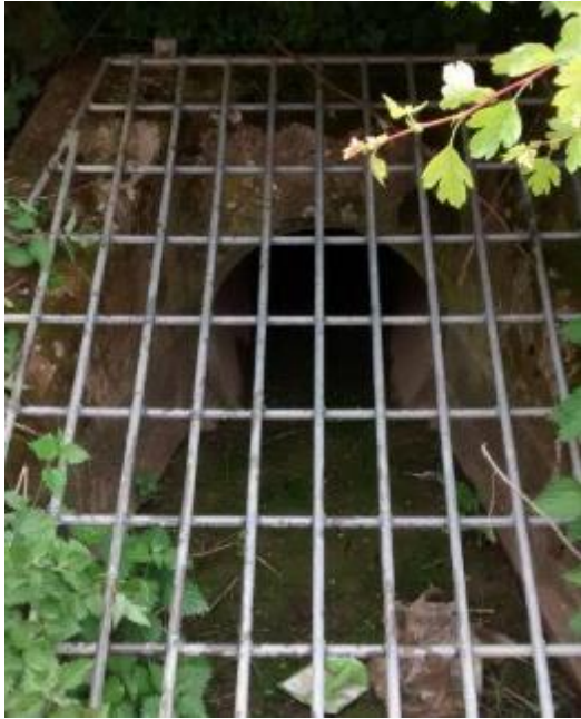
Image 10-19 – B6347 Western Culvert (Inlet)
