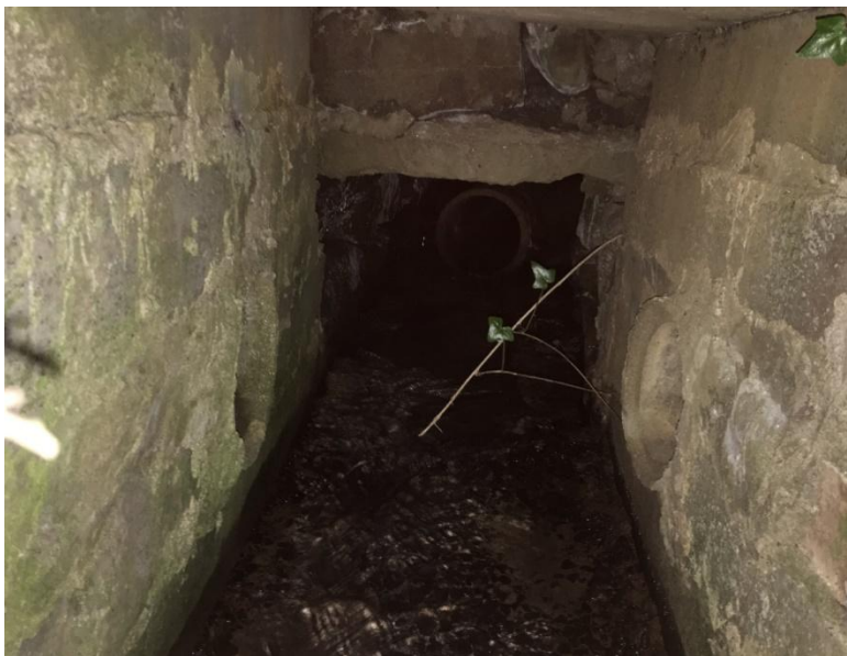
Image 10-16 – Farm Access Track Culvert Along Tributary of White House Burn (Outlet)
