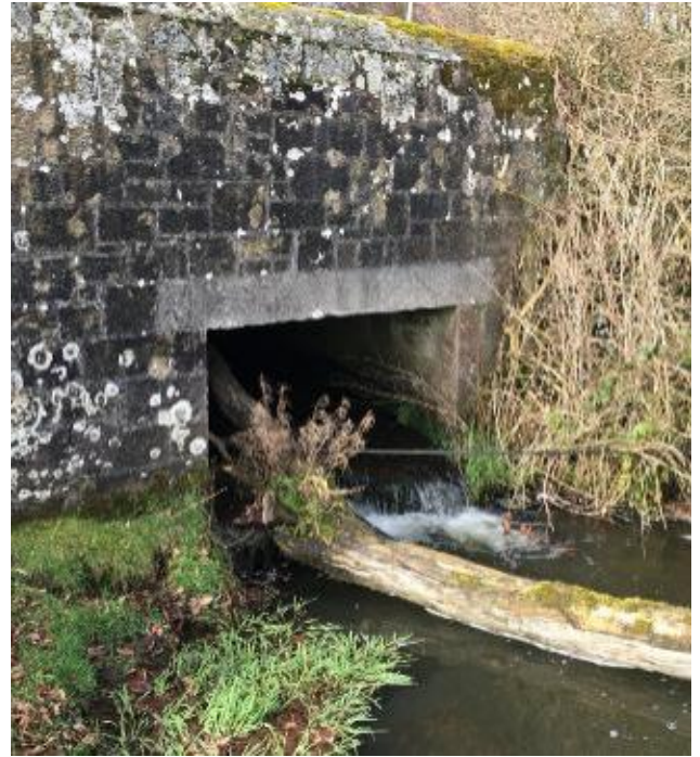
Image 10-31 – Shipperton Bridge (Outlet)
