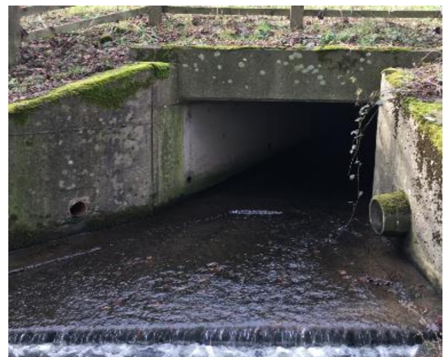
Image 10-29 – Shipperton Burn A1 Culvert (Outlet)
