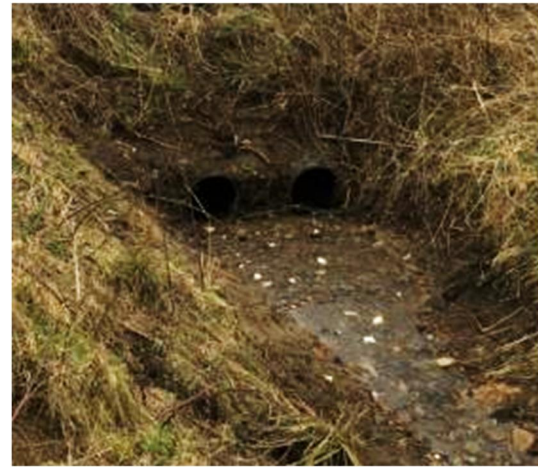
Image 10-12 - Farm Access Culvert 1 Inlet
