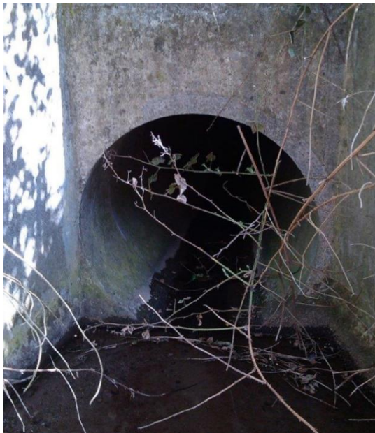
Image 10-3 - Denwick Burn A1 Structure 4 Culvert Inlet
