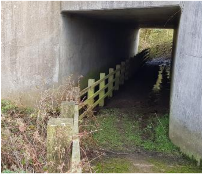
Image 10-14 – White House Burn A1 Culvert (Outlet)
