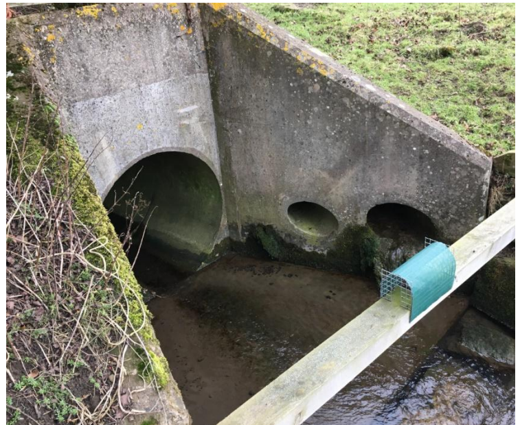
Image 10-4 - Denwick Burn A1 Structure 4 Culvert Outlet
