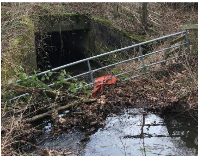
Image 10-28 – Shipperton Burn A1 Culvert (Inlet)
