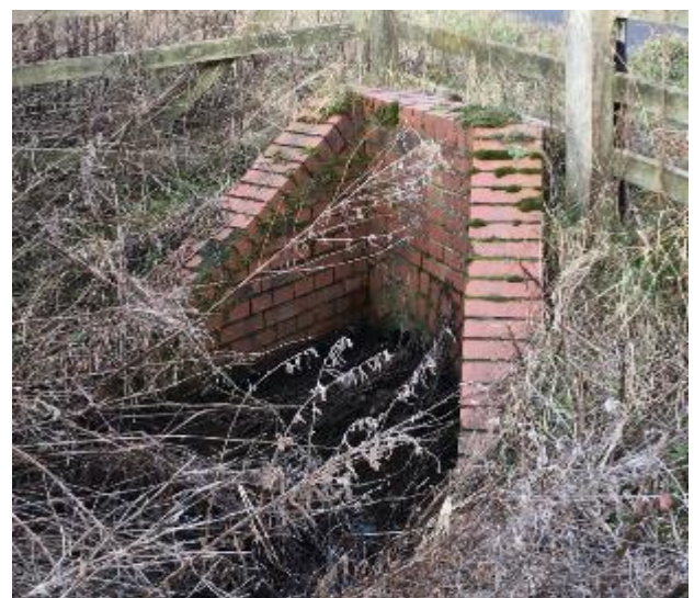
Image 10-22 – B6347 Eastern Culvert (Inlet)
