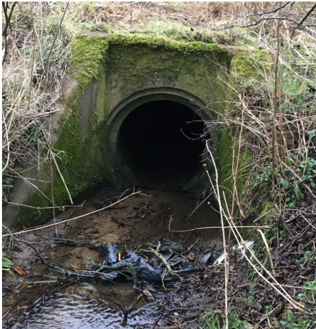
Image 10-7 - Denwick Burn A1 Structure 3 Culvert Inlet
