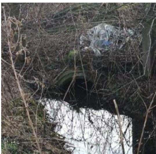
Image 10-21 – Small Access Track Culvert (Outlet)
