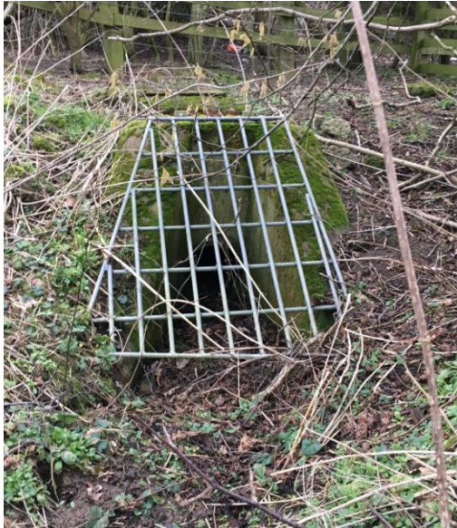
Image 10-8 - Denwick Burn A1 Structure 2 Culvert Inlet
