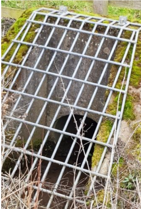
Image 10-2 - Heckley Fence Culvert Inlet
