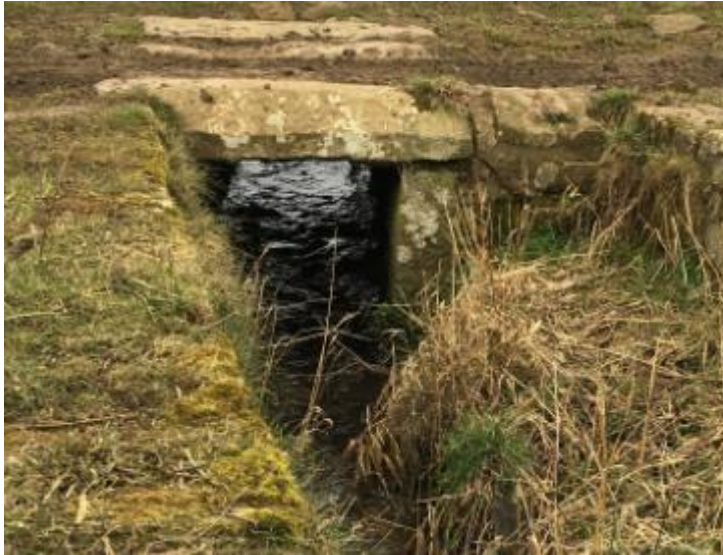
Image 10-5 - Public Right of Way Denwick Burn Crossing
