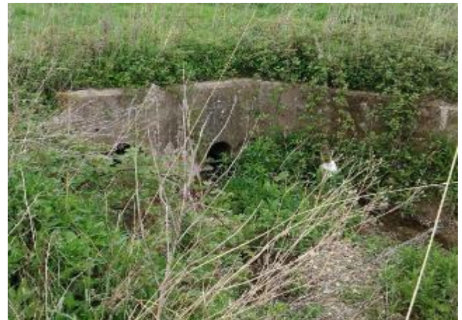
Image 10-10 - Farm Access Culvert 2 Outlet
