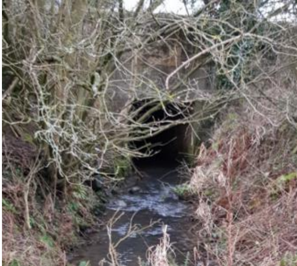
Image 10-17 – Culvert Underneath the B6341 (Inlet)
