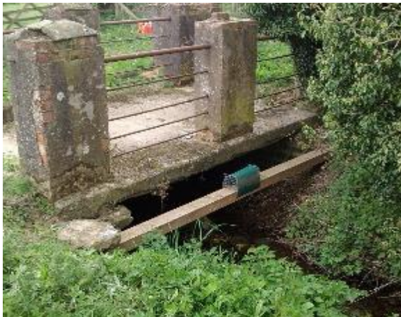
Image 10-9 - Farm Access Culvert 2 Inlet
