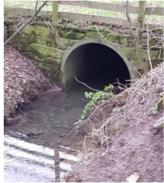
Image 10-15 – White House Burn Field Access Culvert (Outlet)
