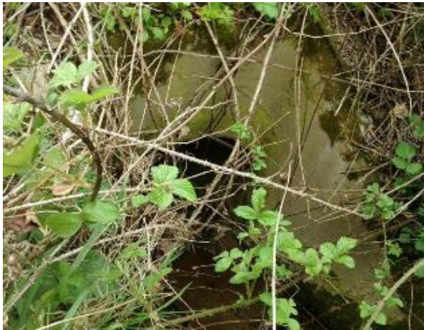
Image 10-11 - Denwick Burn A1 Structure 1 Culvert Inlet
