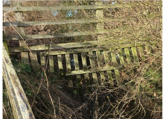
Image 10-24 – Debris Fence along Unnamed Western Tributary of Kittycarter Burn
