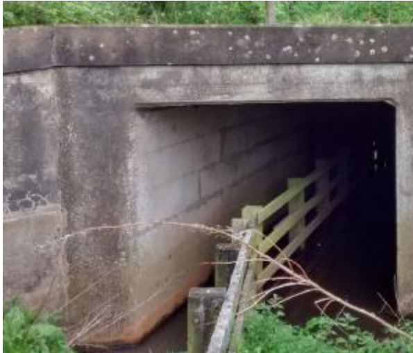
Image 10-23 – Western Tributary of Kittycarter Burn Culvert Underneath A1 (inlet)
